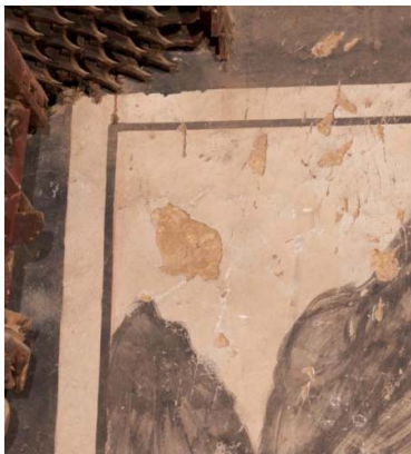
Figure 6 Coating shedding (No.26 excerpt)
