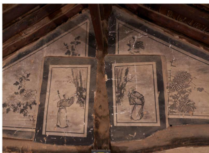
Figure 2 Mural cracks on the upper part of the east gable (No.9)
